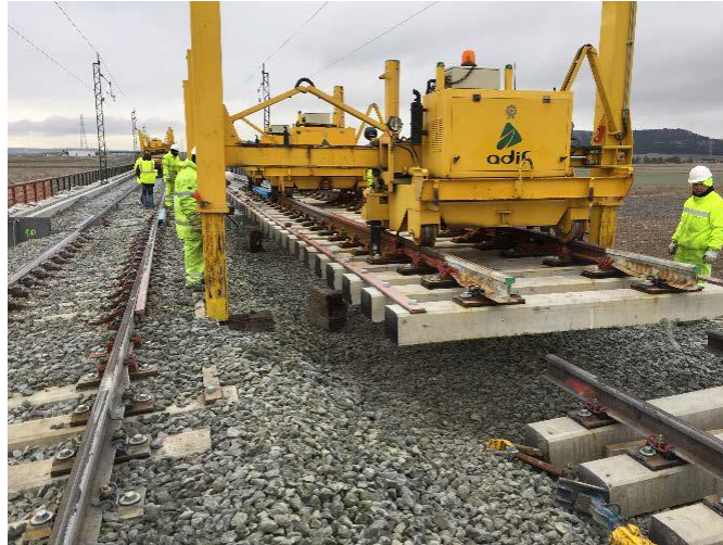
Plate 4.2 Rail panel handling machine
