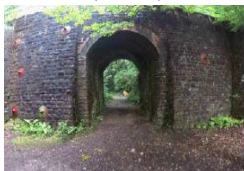
An example of bridge strengthening using tie bars and pattress plates
