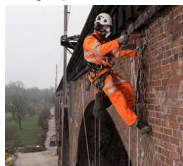
An example of bridge strengthening using roped access
