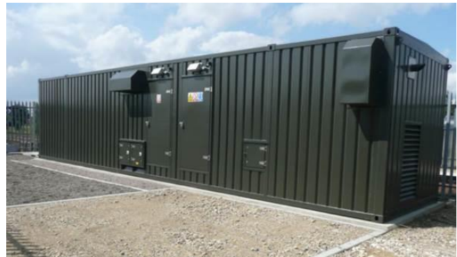
Plate 4.3: Example of a principal supply point
